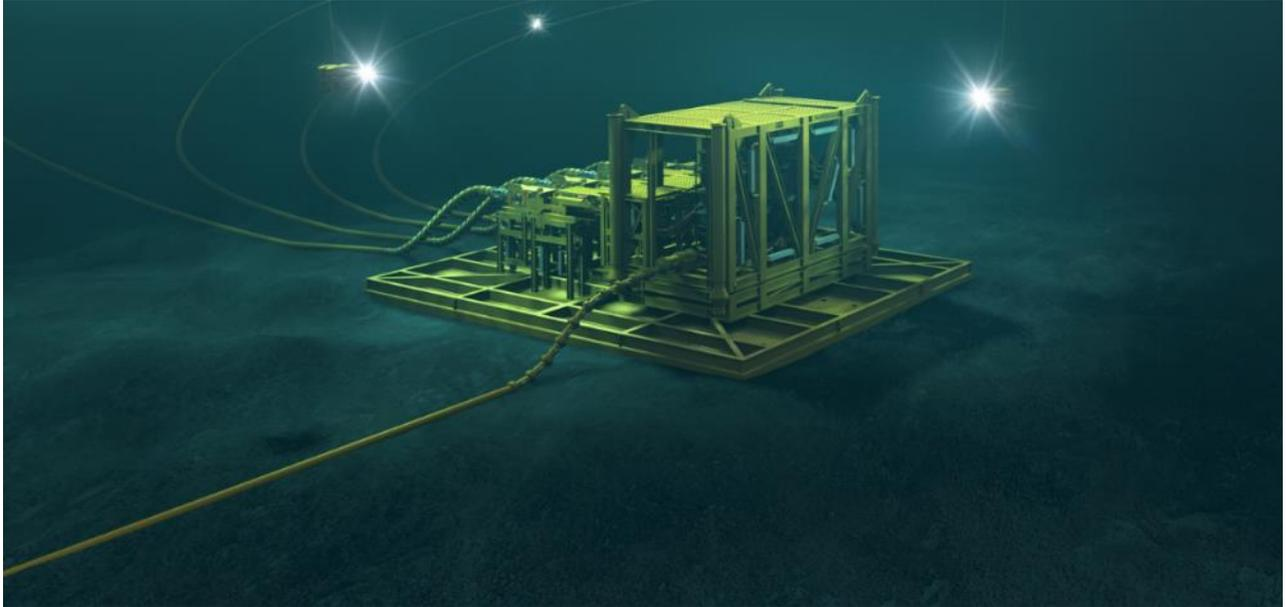
**Figure 8-25: Subsea Transformer Station with incoming cable from shore (front) and outgoing cables to FPSOs (back).
